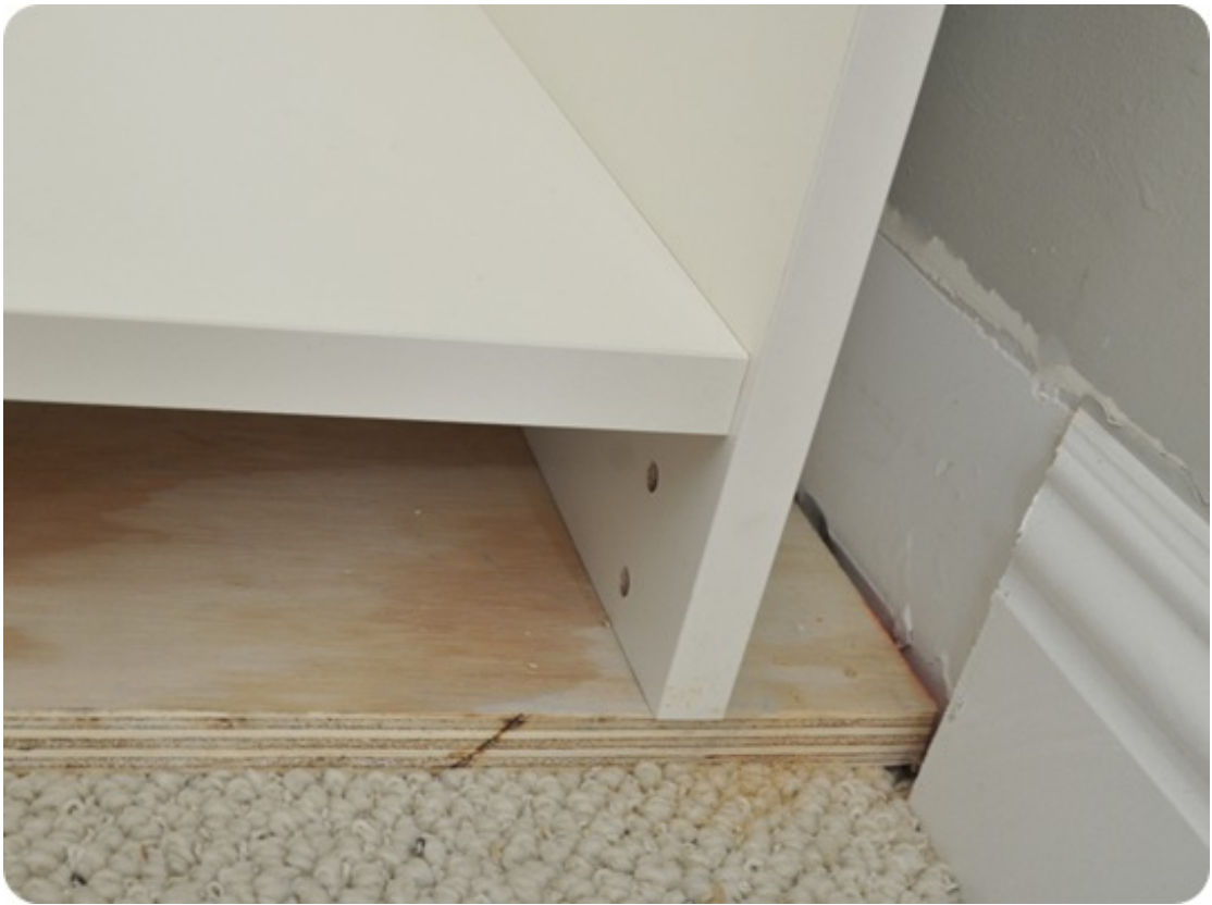
Once the bookcases were elevated, the baseboard trim fit perfectly in front.
