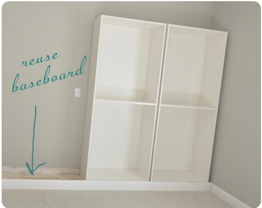
Once the bookcases were elevated, the baseboard trim fit perfectly in front.
